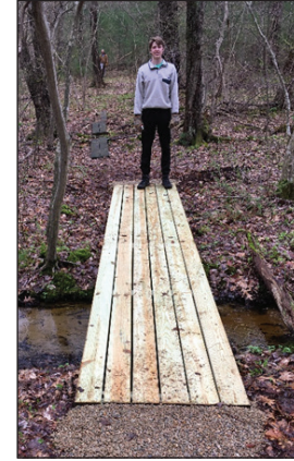
Hesselman shown with boardwalk as it neared completion.
